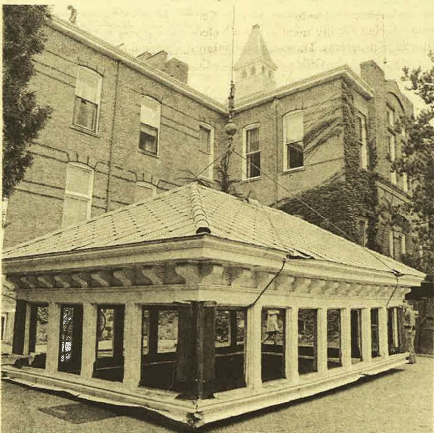
Raising the roof
