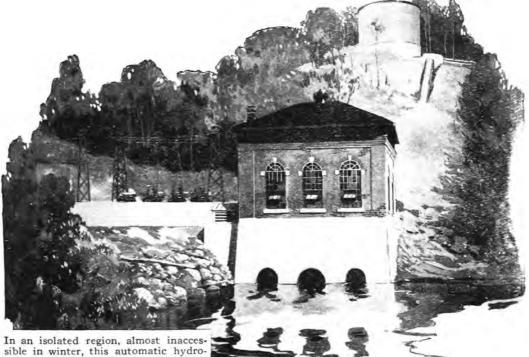
In an isolated region, almost inaccessible in winter, this automatic hydroelectric plant of the New England Power Company on the Deerfield River starts, protects and stops itself.
