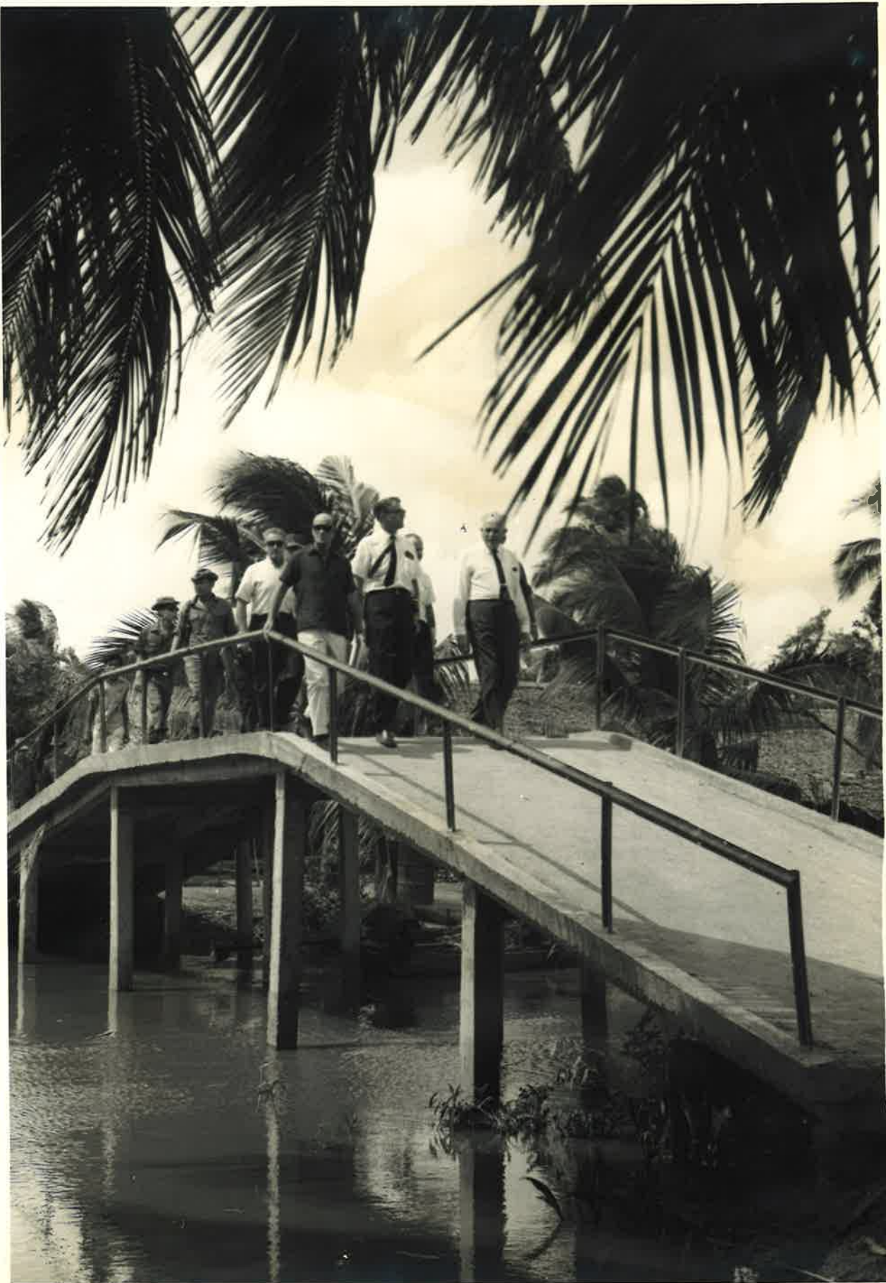
Inspecting self-help projects in the Mekong Delta with Director MacDonald, Dr. Hannah was impressed by this foot bridge financed in part by USAID, the Government of Vietnam, and several villages in the area that contributed manpower and money toward its completion. 1-5 May 69
