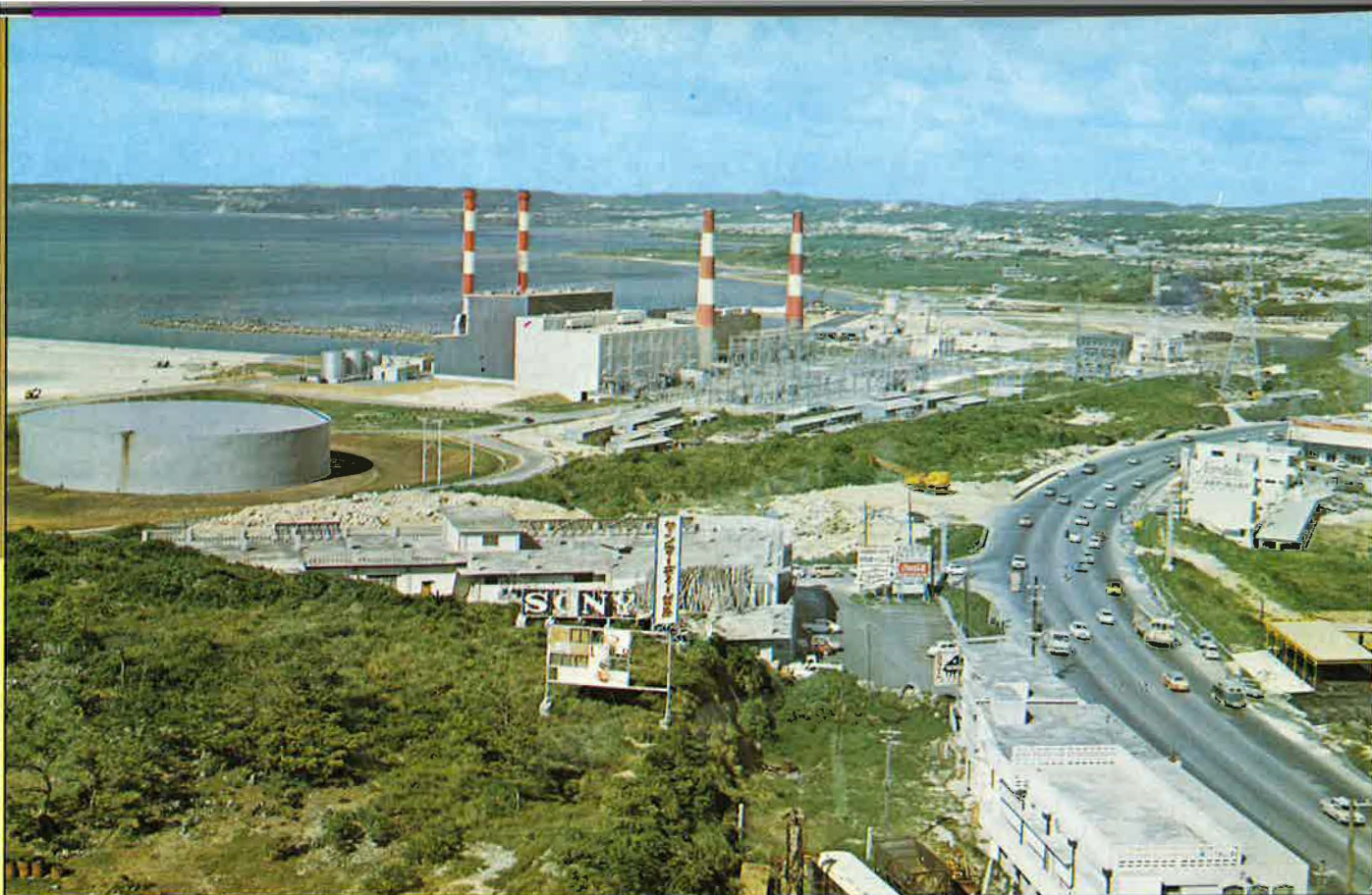
The Machinato Powerplant on Okinawa produces 170,000 kw. of electrical energy with two turbine generators. Its cost was $20.6 million.
