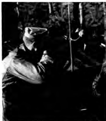
NO MORE FROSTBITE: John V. Polomsky demonstrates his cold weather adapter which allows soldiers to fire rifles with their hands encased in warm, heavy gloves.
